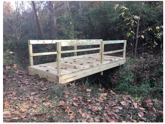
(Top) Timber is carried in on foot on a steep ATV trail across Sparksville easement donor John Howard's property; 16-foot 2x12s are heavy! The bridge spans a steep-sided creek, with nasty slippery vertical banks. (Middle) Students Noah, Brendon, Justin and Mary learn how to build a box, wrangle it across the creek, then insert stringers for this very sturdy bridge. Up-
