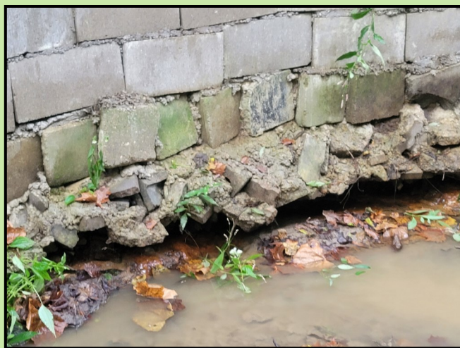
Undermining of the Retention Wall Summer 2022
